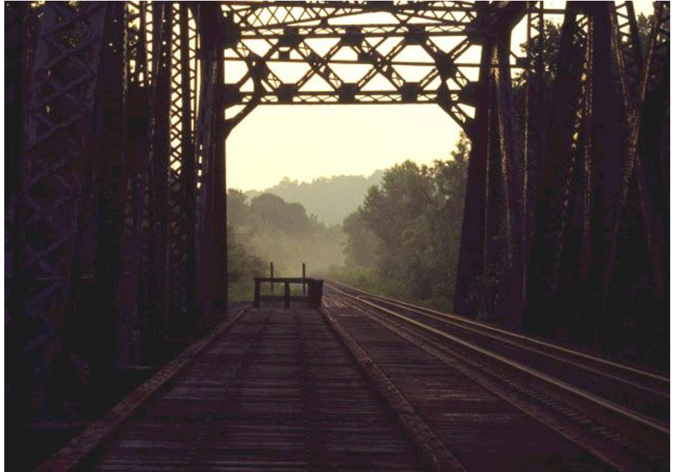
RR Bridge near Barboursville, by F. Huff
